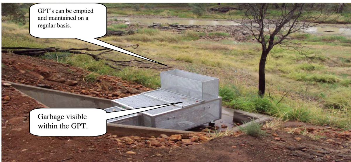
Gross Pollutant Trap in Weir Park near the Brewarrina Fish Traps.
